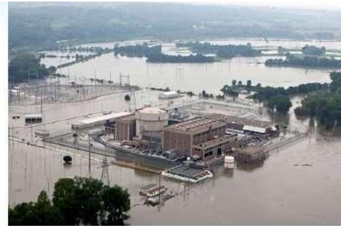
Fort Calhoun plant on June 16, 2011 during the 2011 Missouri River Floods: vital buildings were protected using water-filled perimeter "flood berms" https://energynews.us/2020/08/31/report-climate-risks-compound-financial-challenges-for-midwest-nuclear-plants/
