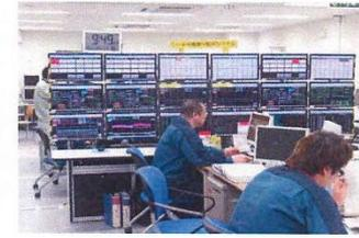
Plant parameters, including RPV and PCV temperatures, are monitored continuously 24 hours a day.
