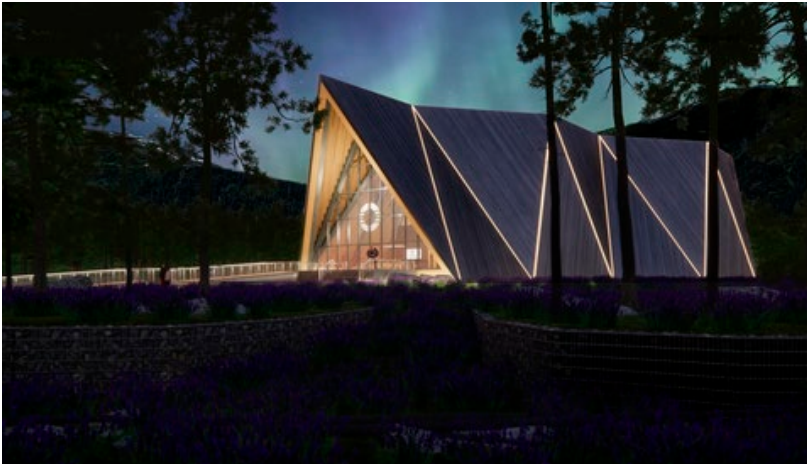
Oklo's Aurora powerhouse
