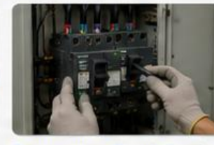
Penggantian Circuit Breaker
