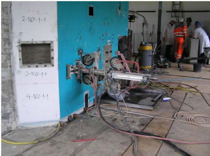
Cutting the four experimental channels
