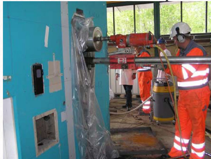
Channel being drilled out
