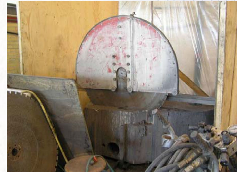
Circular saw cutting away the activated inner slab
