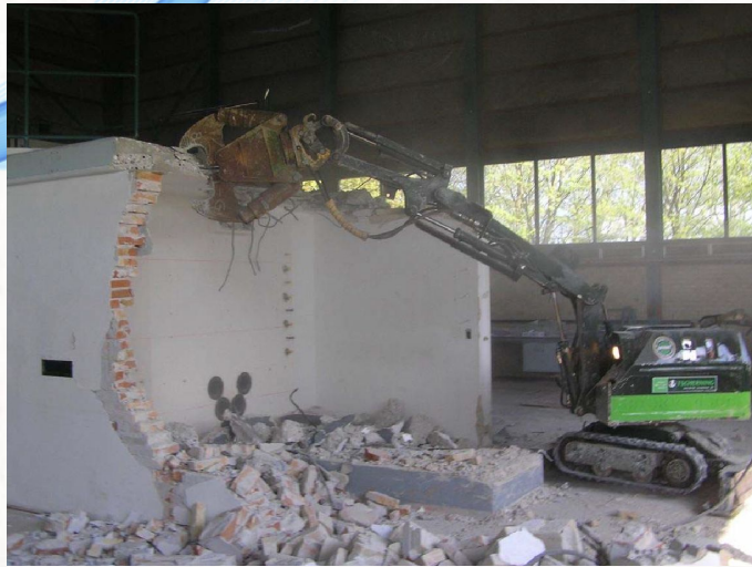
Demolition of the control rod house
