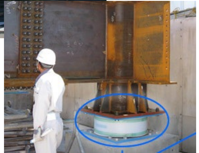
Seismic isolation structure (quake-adsorbing structure) 20
