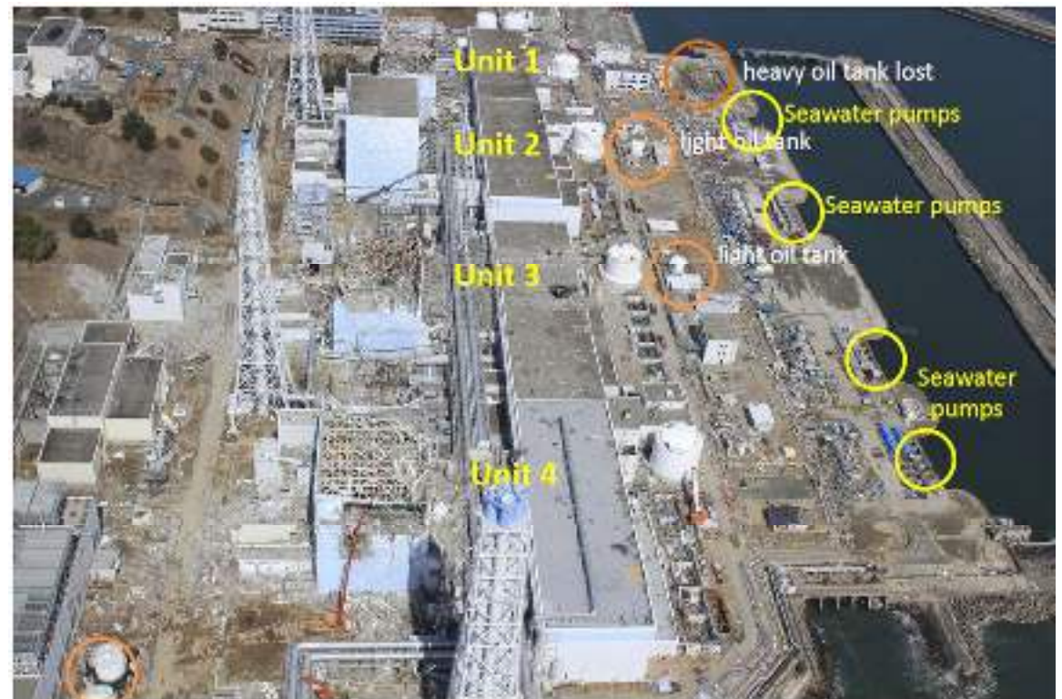
light oil tanks
