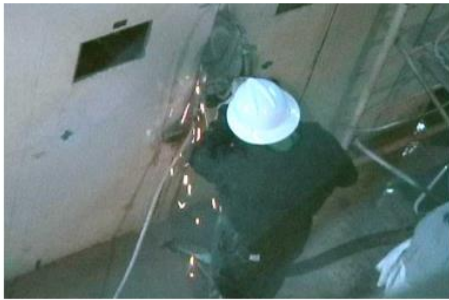
Figure 30. Scoring the Concrete
