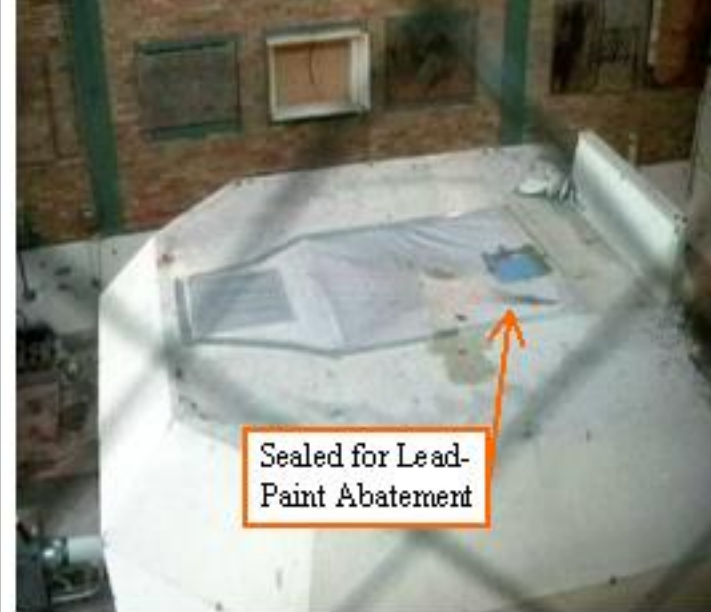
Figure 25. Paint Removal in Progress
