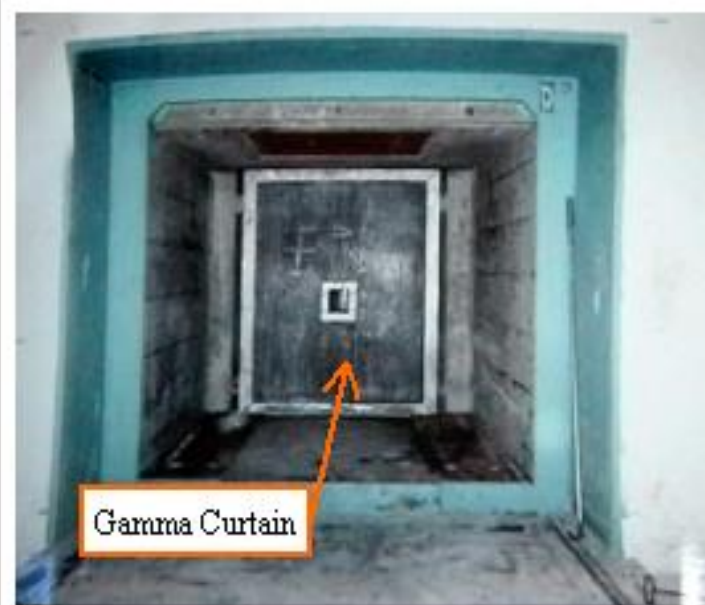
Figure 15. Graphite Removal Completed
