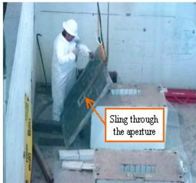
Figure 16. Aluminium Frame Removal
