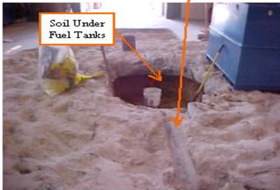
Figure 54. Activated Floor/Soil Removal
