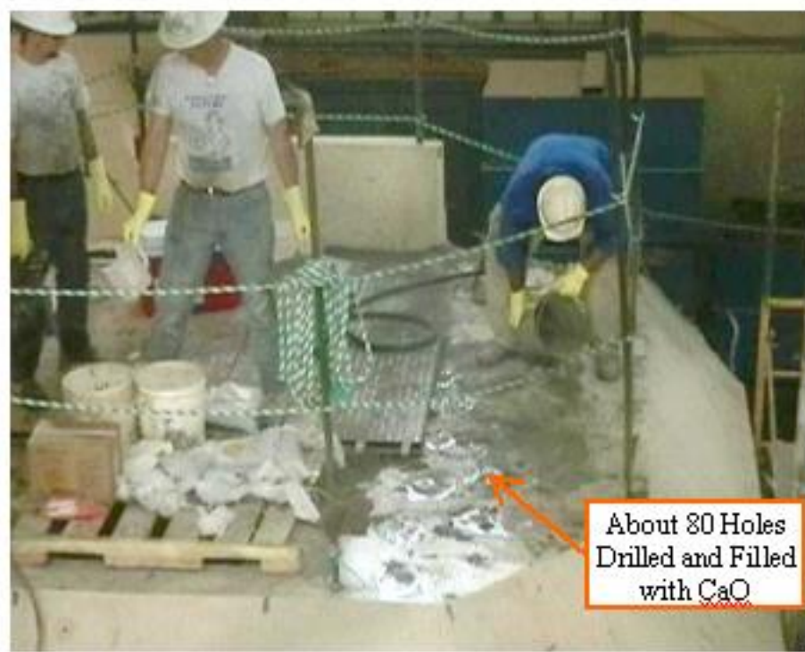
Figure 36. Holes being filled with CaO
