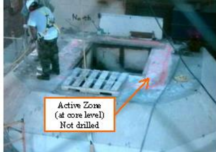
Figure 34. Drilling – 20 minutes per hole
