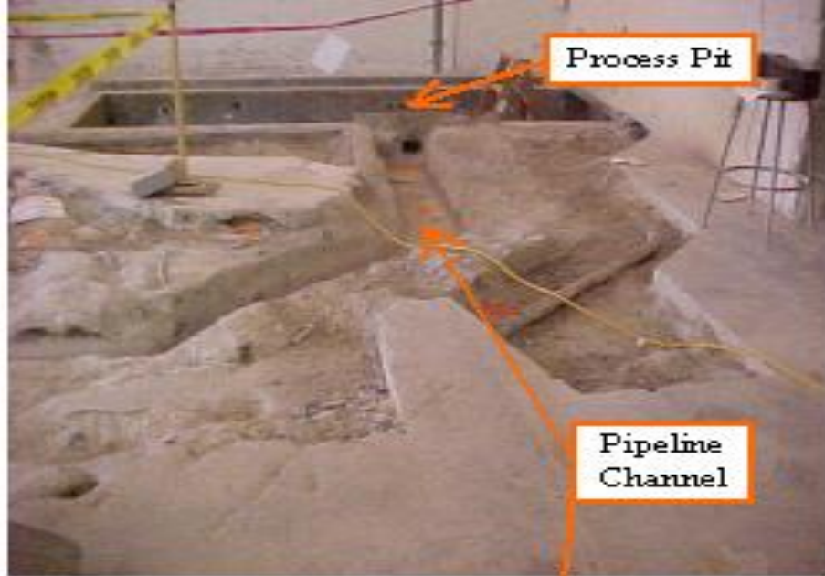
Figure 52. Pipeline Pit
