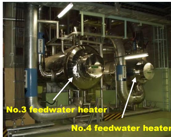
Before dismantling activity
