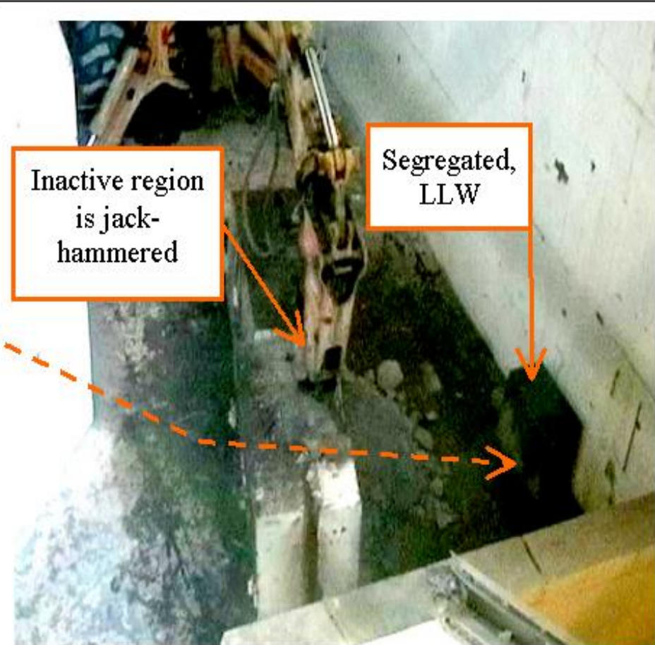
Figure 11. Active Plug Segregation
