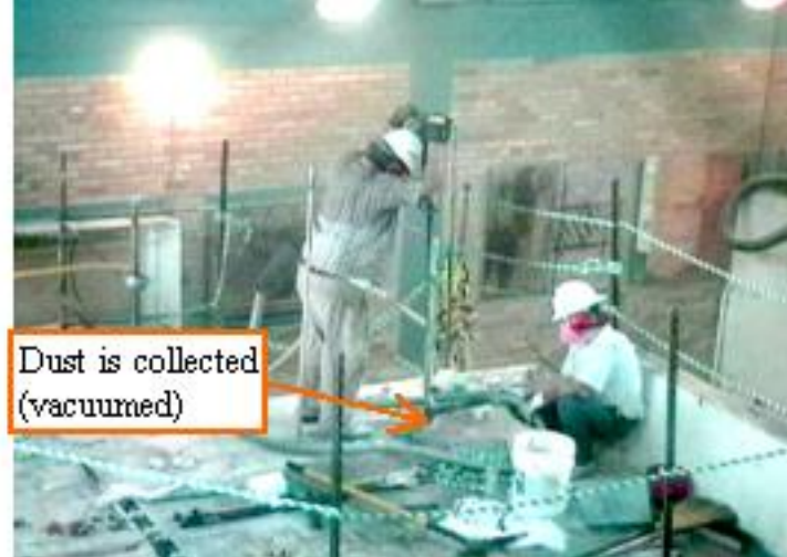
Figure 35. Drilling and Vacuuming
