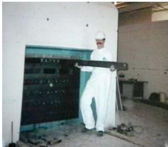
Figure 12. Graphite Removal by Hand
