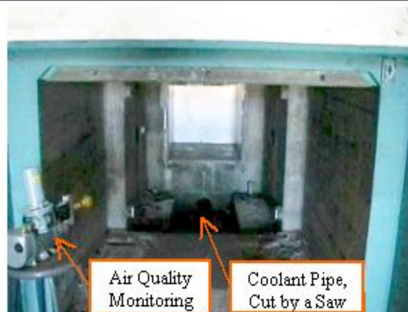
Figure 21. Components Removed
