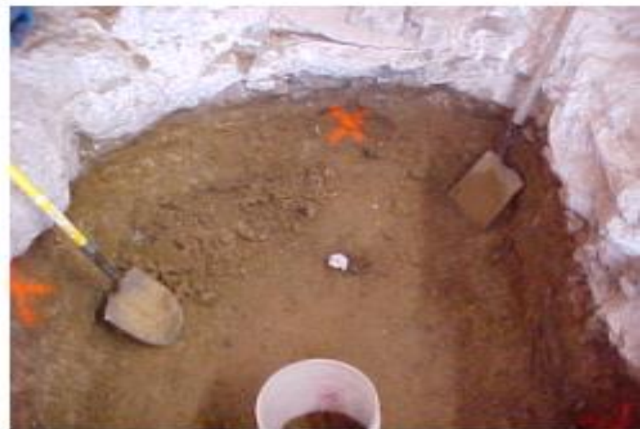
Figure 55. Activated Zone Excavated
