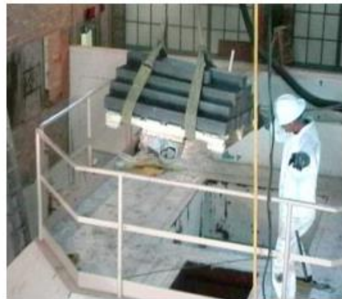
Figure 13. Graphite Removal by Crane
