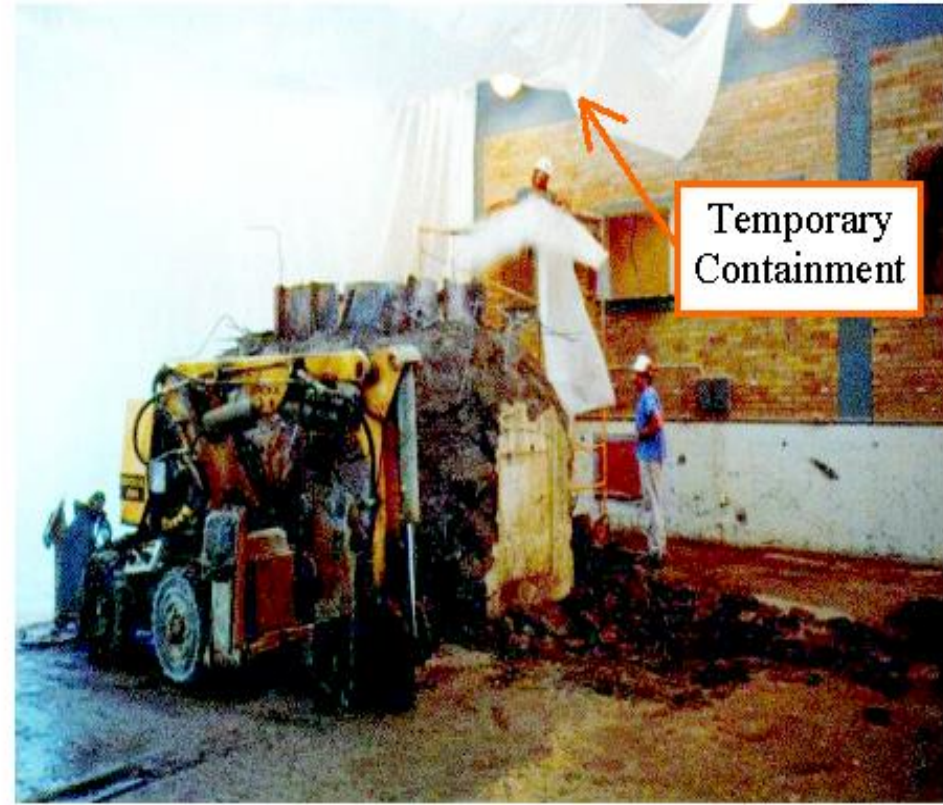
Figure 45. Day 4 – Containment Set-up
